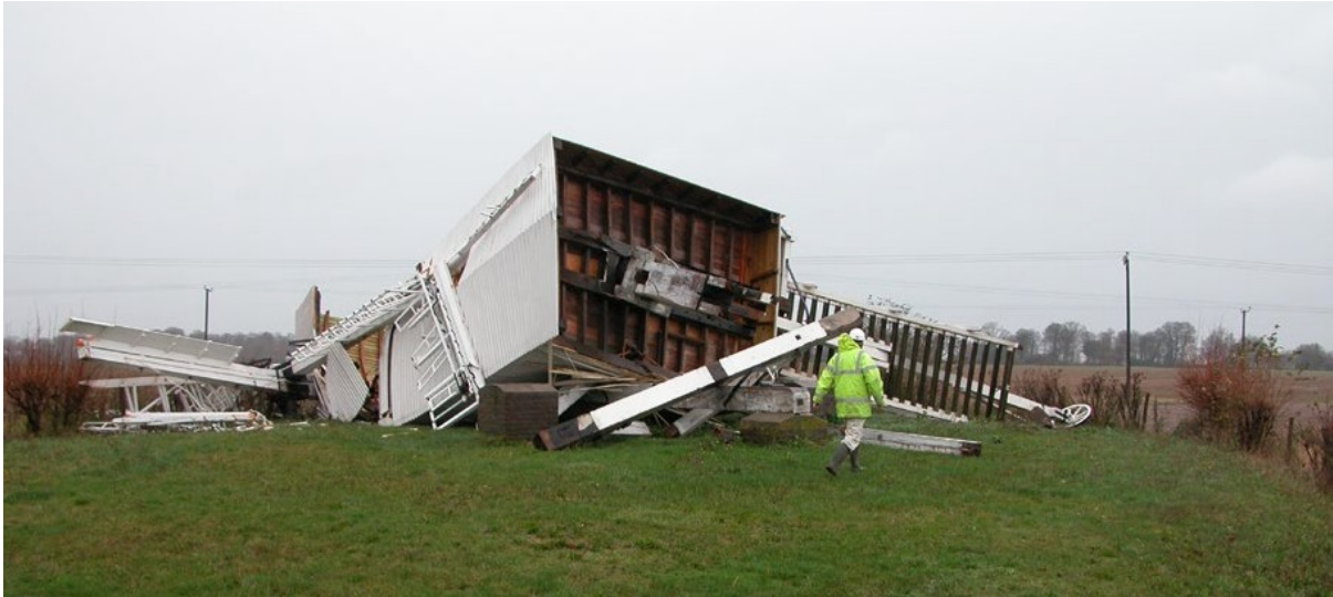
Figure 6 Chillenden windmill, blown down in 2003, now re-built.
